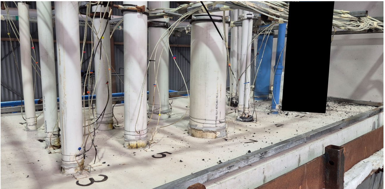
Appendix Figure C-8: Penetrations 1-13, unexposed side at 180 minutes.
