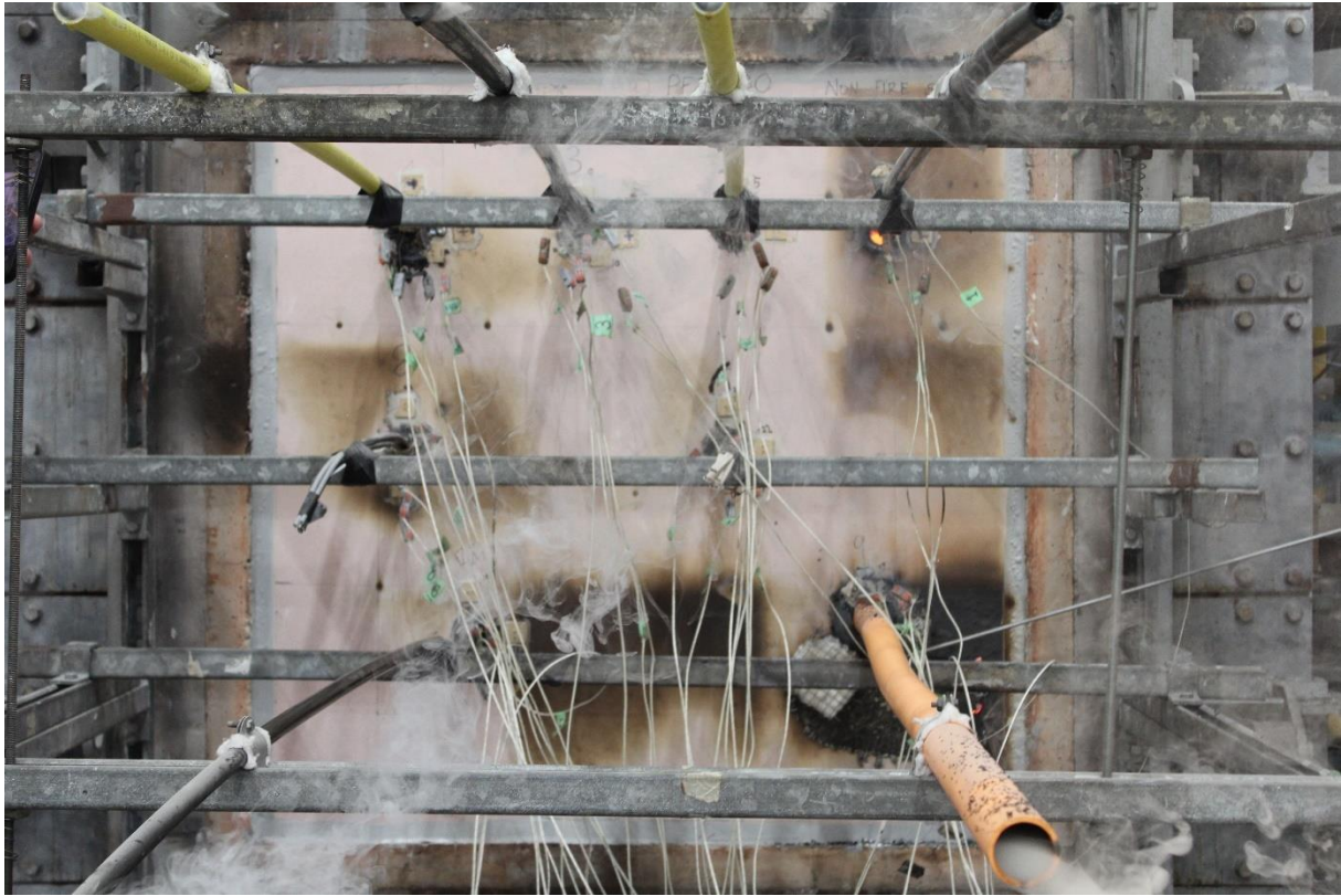
Figure 43 – Unexposed face at 90 minutes
