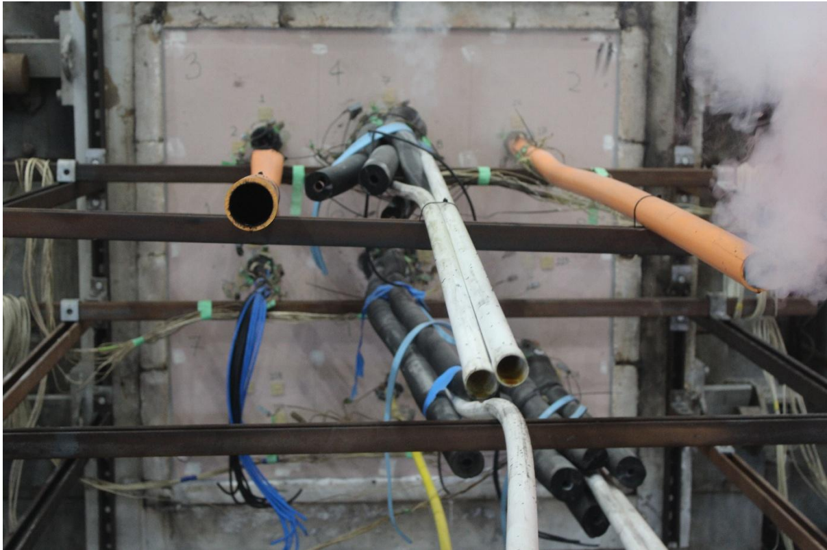
Figure 32 - Unexposed face at 90 minutes
