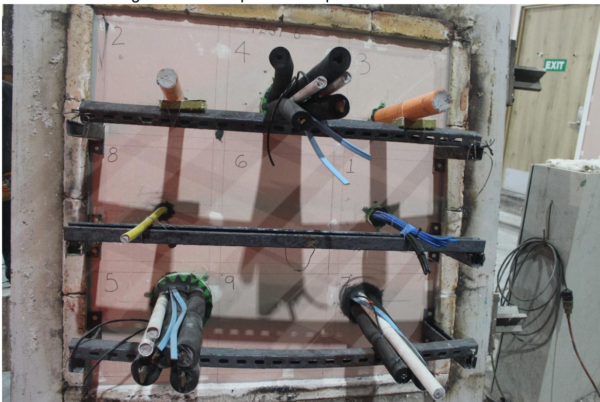
Figure 23 - Exposed face prior to test commencement
